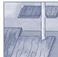
20. If you wish to remove the flooring, just lift the planks a few centimetres and tap along the joint.
